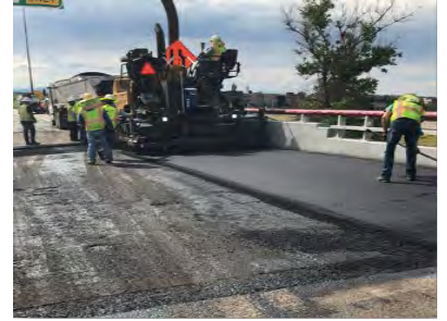
Image: Pavement overlay on the roadway
