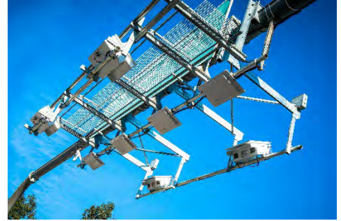
Image: Overhead Tolling Detection System
