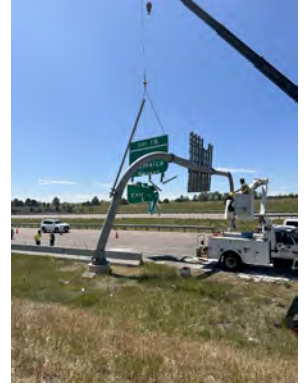
Image: Crew Replacing Road Sign
