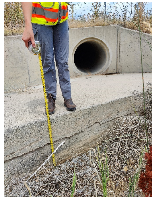
Figure 2-4 – Box 2ft of scour at inlet of culvert near TPE (SB)
