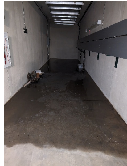
Figure 2-8 – TPD – Standing water in tunnel area.
