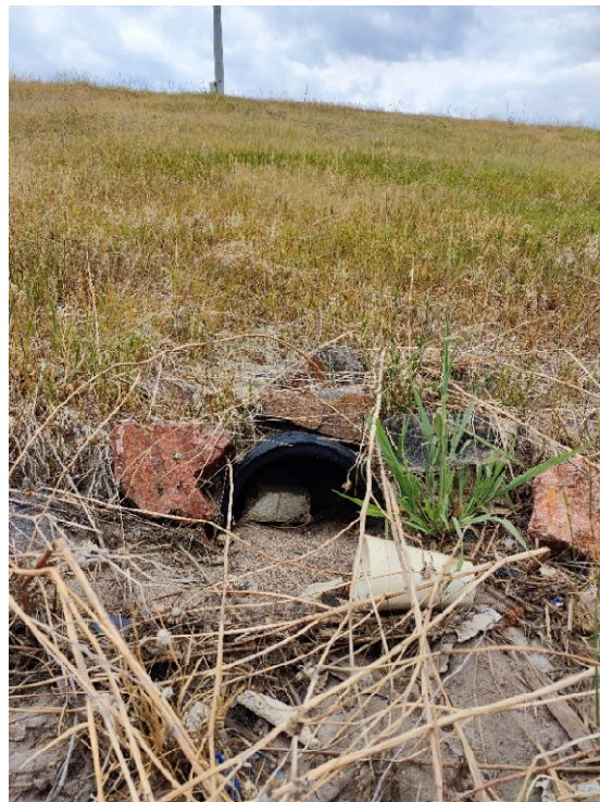
Figure 2-13 – Trash and sediment buildup at EP outlet, SW of S Parker Rd Bridge (NB)
