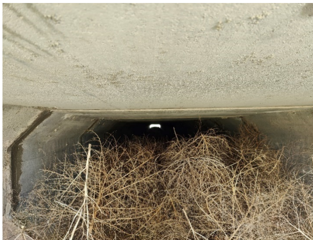
Figure 2-3 – Box Culvert with significant tumbleweed build-up at MP 37.5
