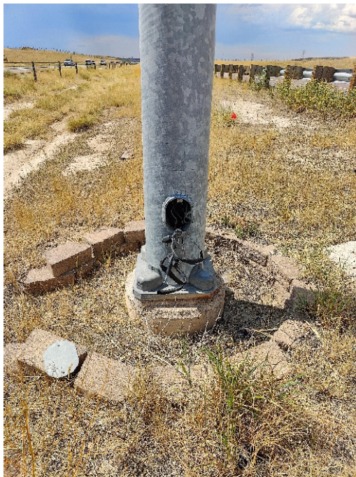
Figure 2-1 – Open access panel with wires exposed, median at Toll Plaza B
