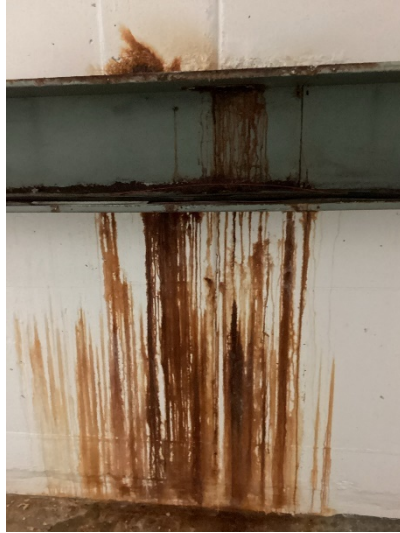
Figure 2-7 – TPA – Water damage
