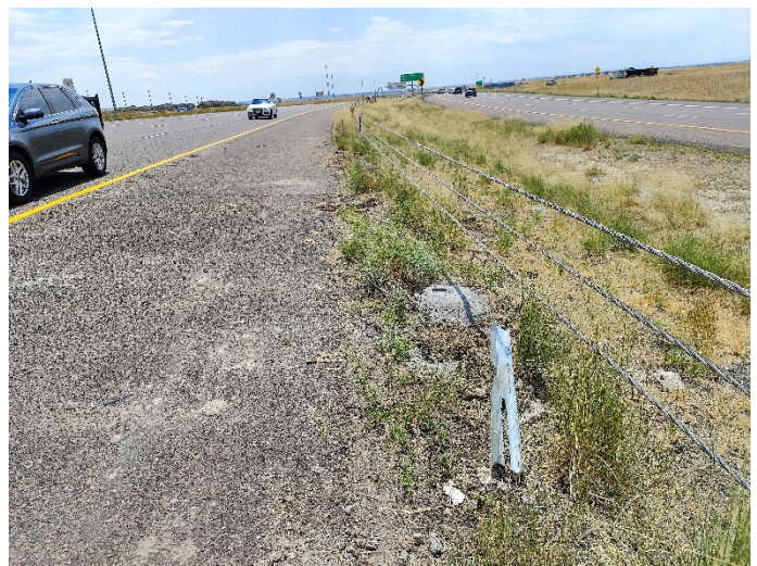
Figure 2-6 – Stretch of damaged cable rail in median near 96 th Avenue
