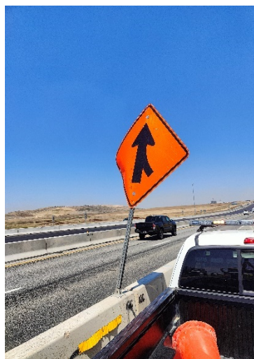
Figure 2-10 – Bent sign panel on out-of-plumb pole in work zone
