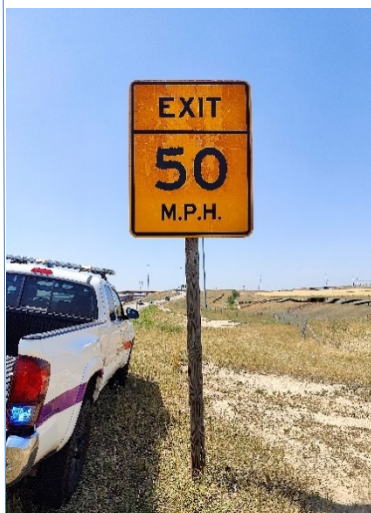
Figure 2-9 – Faded peeling sign near I-25 North Ramp Exit
