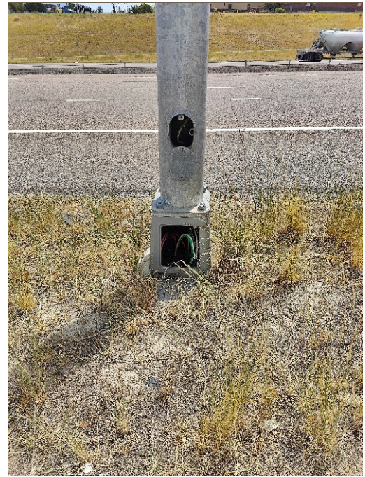
Figure 2-2 – Multiple open access panels, observed at multiple locations
