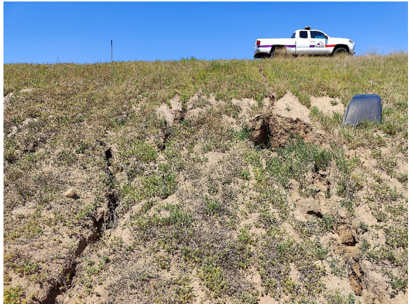
Figure 2-12 – Multiple 12in+ ruts observed on embankment SE of I-76
