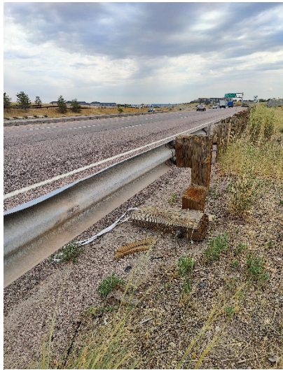
Figure 2-5 – Minor guardrail damage near NB MP1
