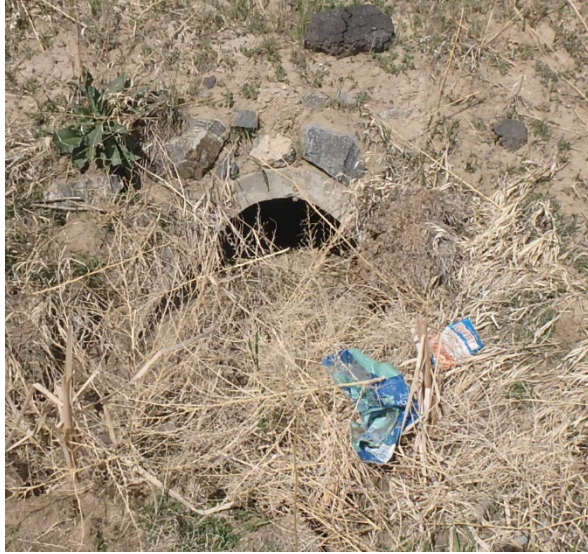
Figure 2-1 – Reinforced Concrete Pipe Flared End with Tumbleweed and Trash Build-Up
