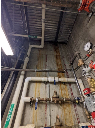
Figure 2-3 – Stain on Basement Wall in Toll Plaza D
