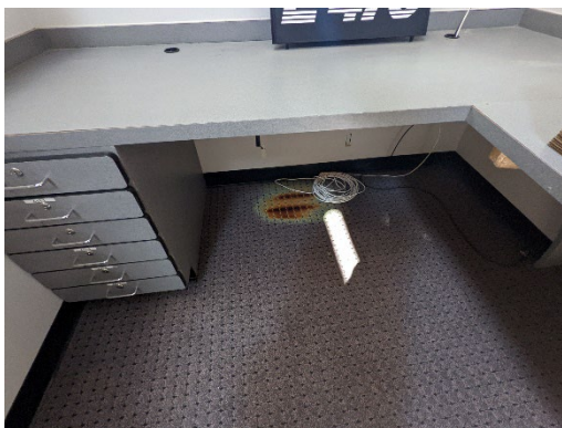
Figure 2-2 – Water Stain on Floor and Ceiling in Toll Plaza A
