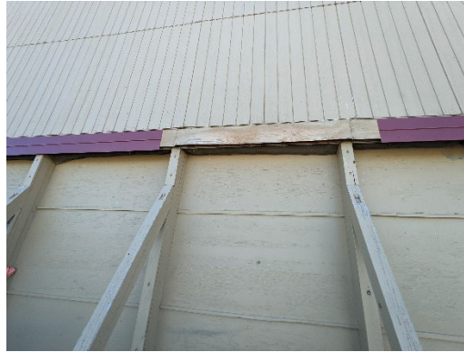
Figure 2-4 – Damage to Plywood Paneling/Sheeting and Missing Cladding on MSS D Exterior
