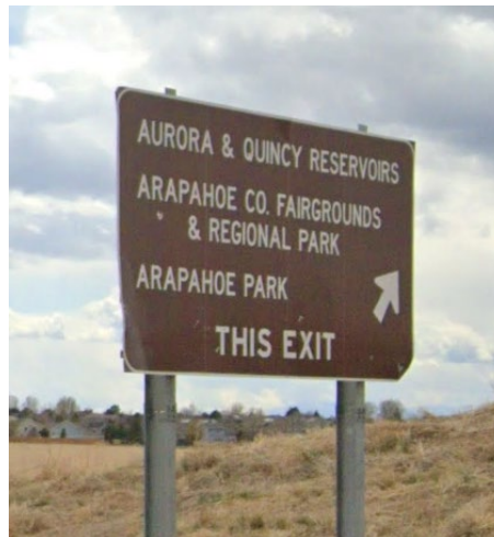
Figure 2-5 – Chipped and Fading Sign SB Before Quincy Ave Off Ramp
