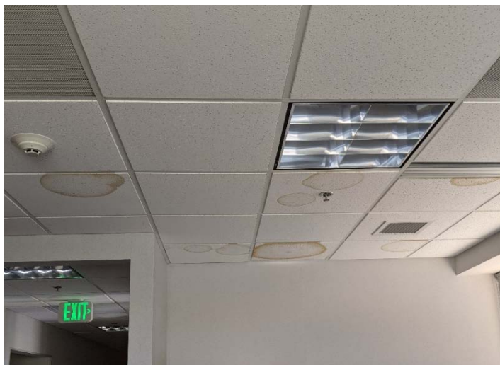
Figure 2-3 - Water Damages and Discoloration to Ceiling
