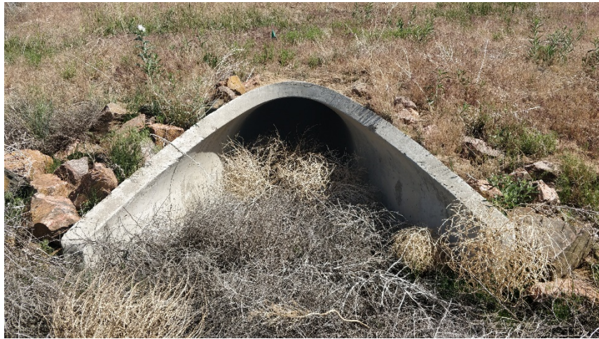
Figure 2-1 – Reinforced Concrete Pipe Flared End with Tumbleweed Build-Up
