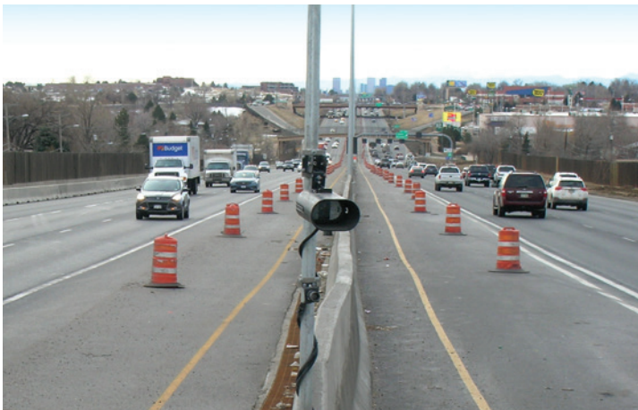
The new I-25 North Express Lanes remained behind barricades as ExpressToll technicians completed tolling equipment installation near 104th Avenue. The downtown Denver skyline is visible in the distance.
