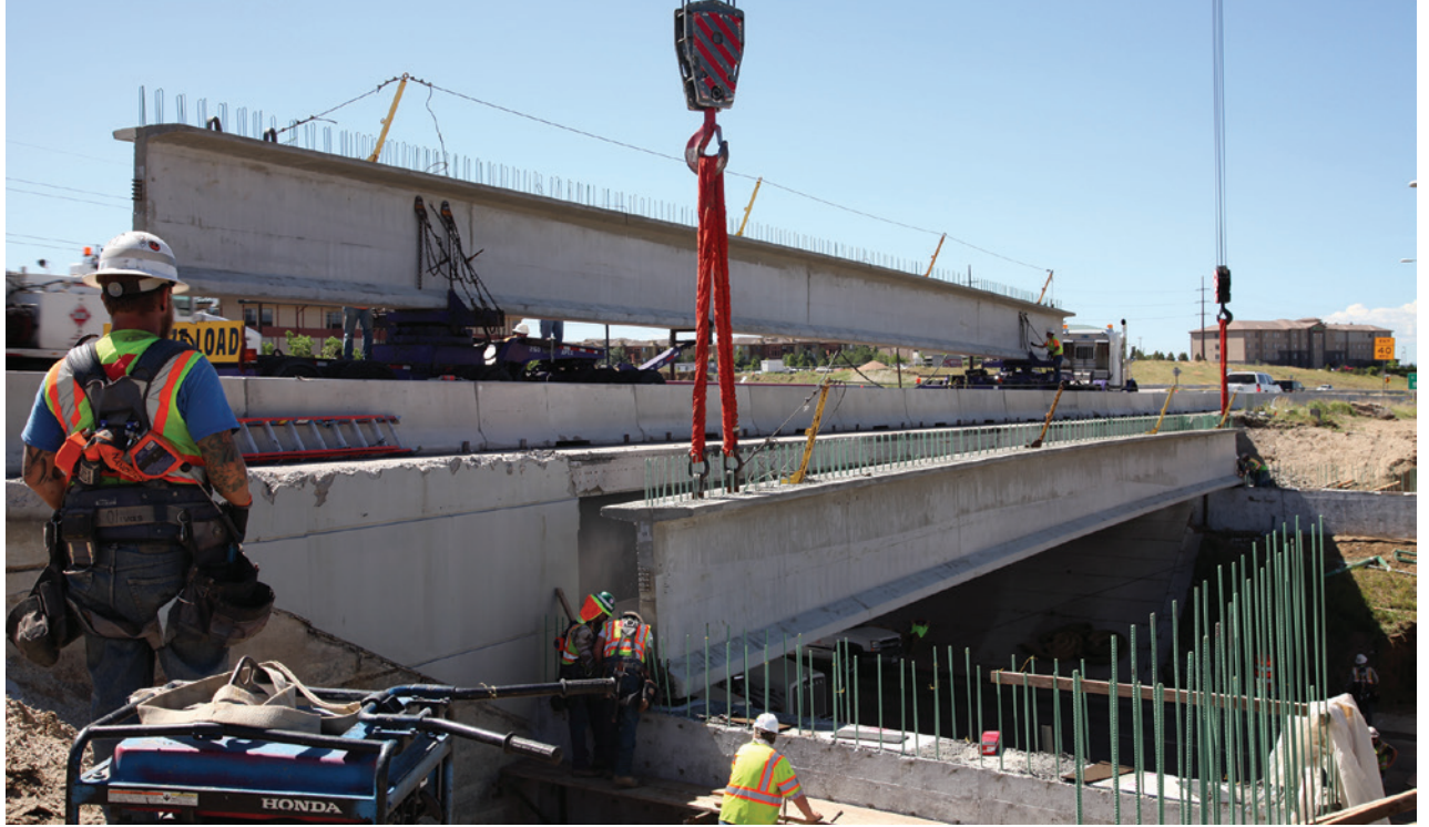
Above right: Placing bridge girders. Eleven bridge structures will be widened to accommodate extra lanes along an eight-mile stretch of E-470. Above left: E-470 Executive Director Tim Stewart leads a pre-construction open house dialogue with residents who live near the tollway expansion project. Left center: On-ramp in the construction area. Bottom left: Widening the way for tollway expansion.
