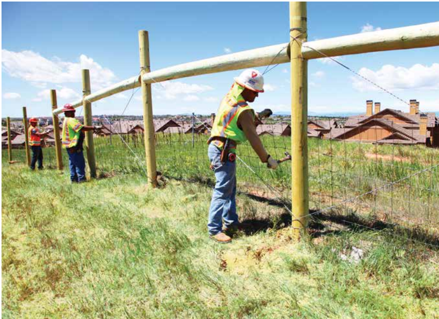
E-470 installed deer fencing to keep wildlife off the highway.
